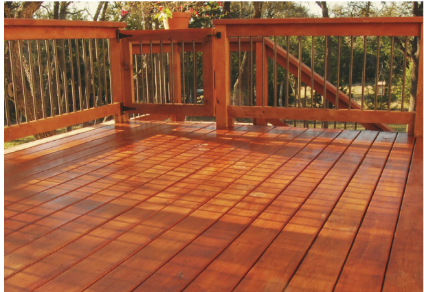
Heat-treated southern yellow pine is also available. The manufacturer recommends coating the decking with Seal It Green Xtreme to help preserve the decking's golden brown color.
