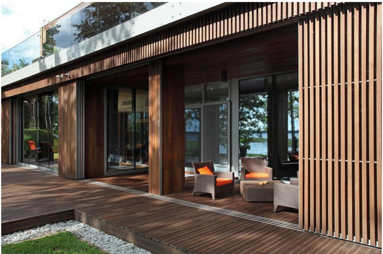
Thermally modified wood's durability and attractive appearance are leading to increased popularity, especially on high-end projects
