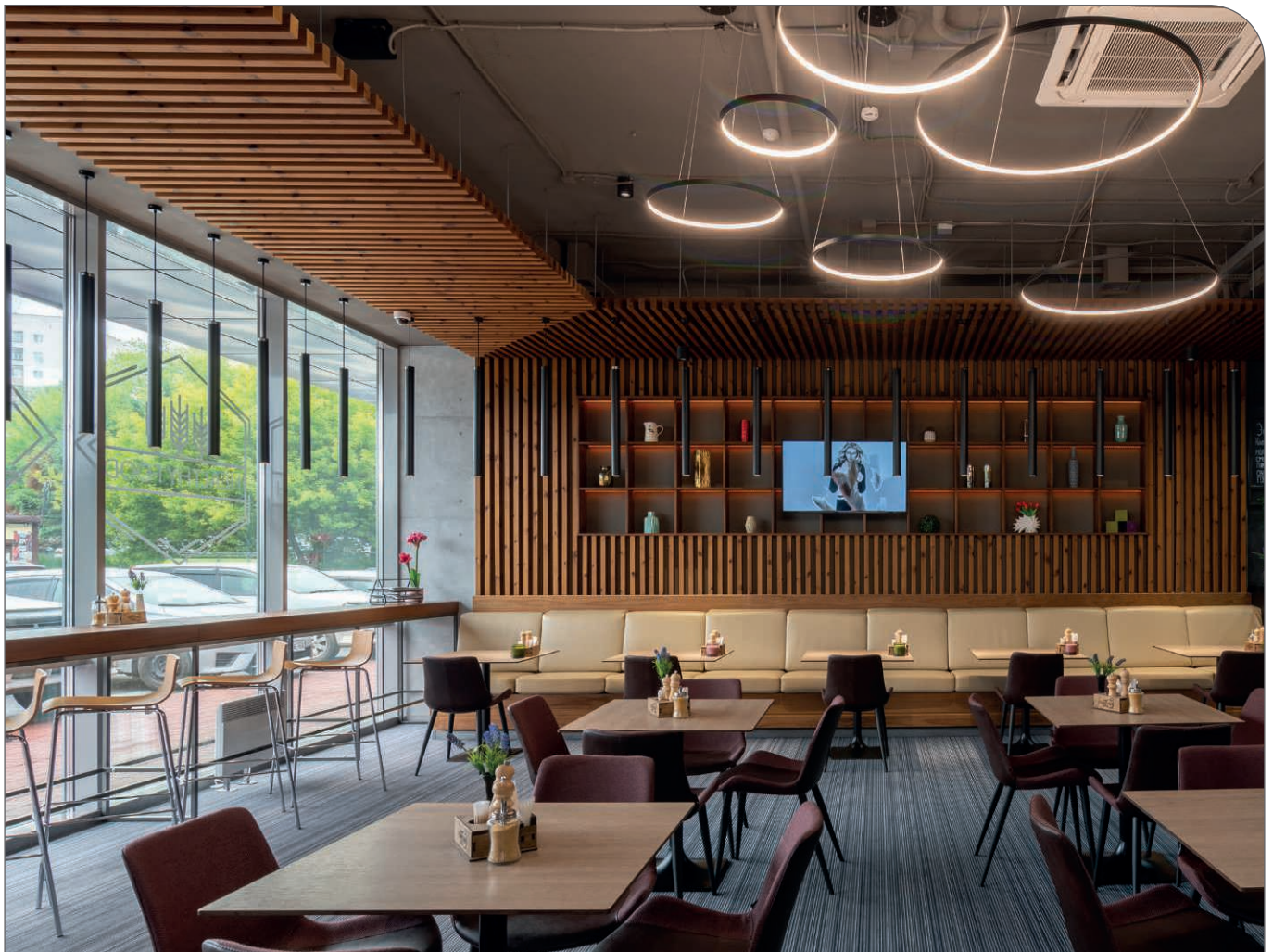
Figure 40. ThermoWood® products used for interior wall cladding in a café in Russia.
