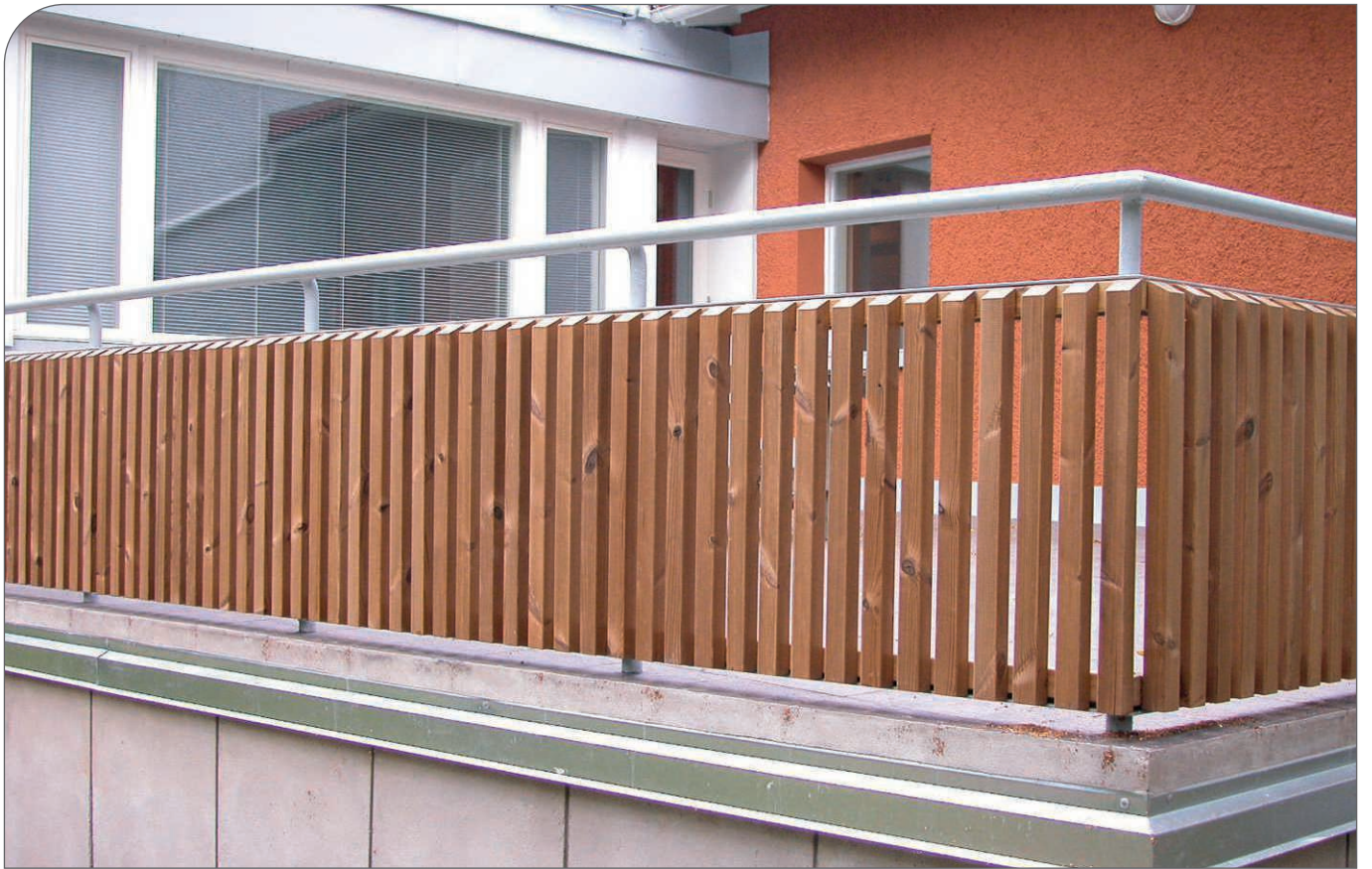
Figure 66. ThermoWood® battens on a balcony railing.
