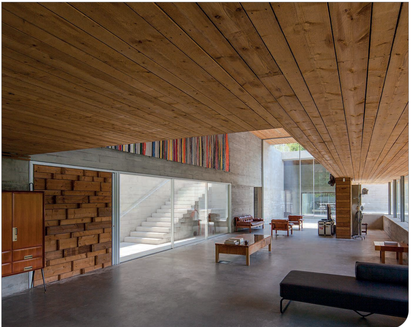
Figure 38. ThermoWood® ceiling in Portugal
