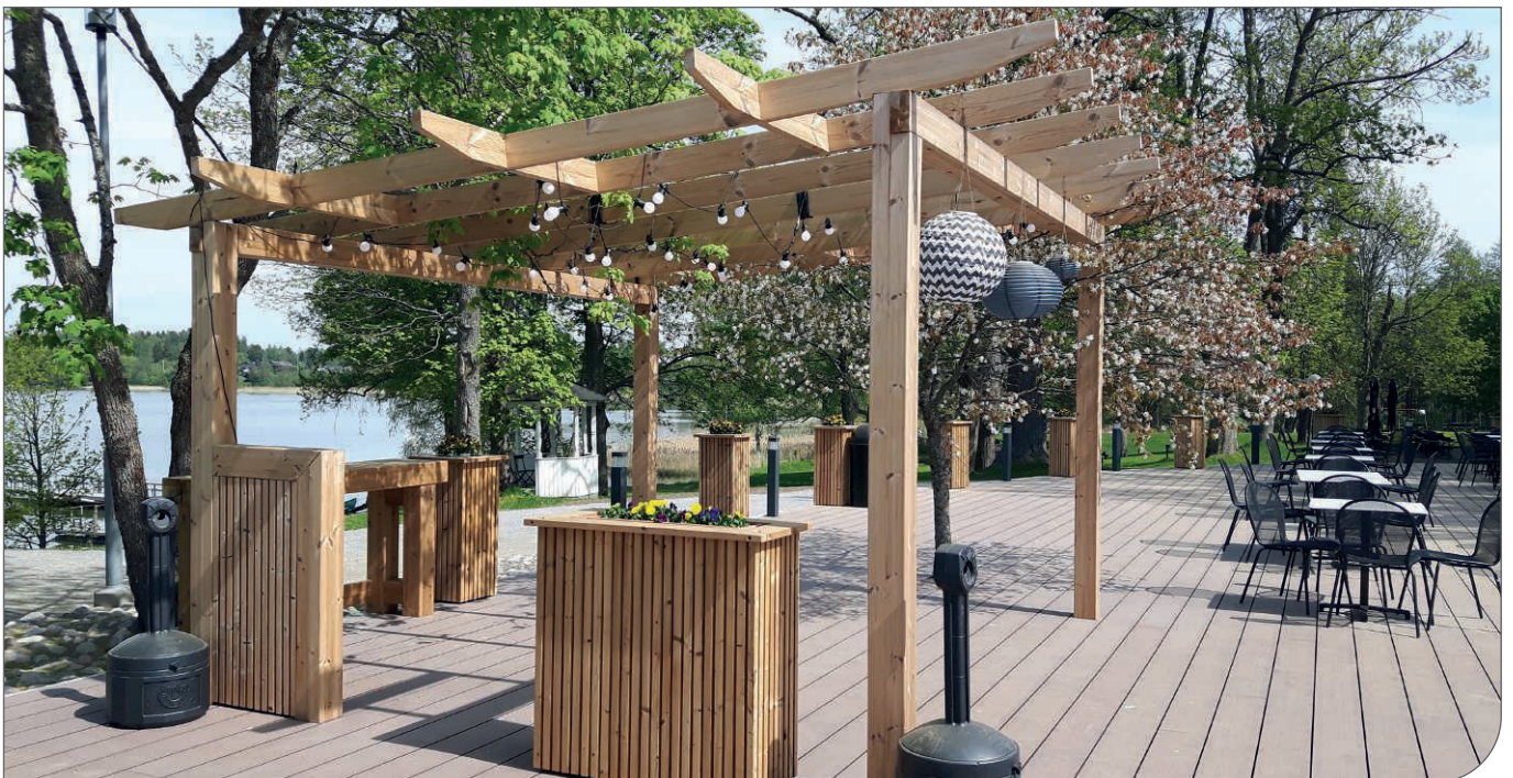
Figure 33. ThermoWood® glue beams in pergola structure
