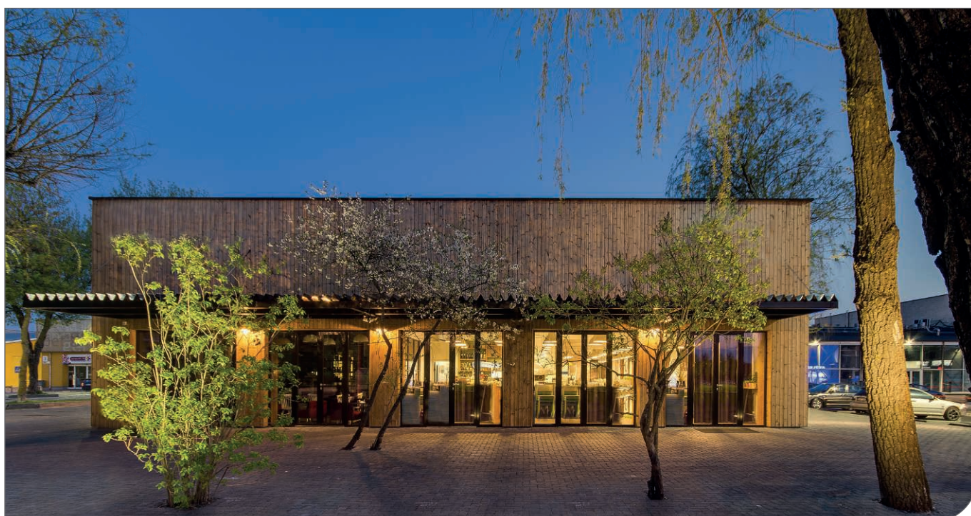
Figure 59. ThermoWood® exterior wall cladding on a Lithuanian restaurant.
