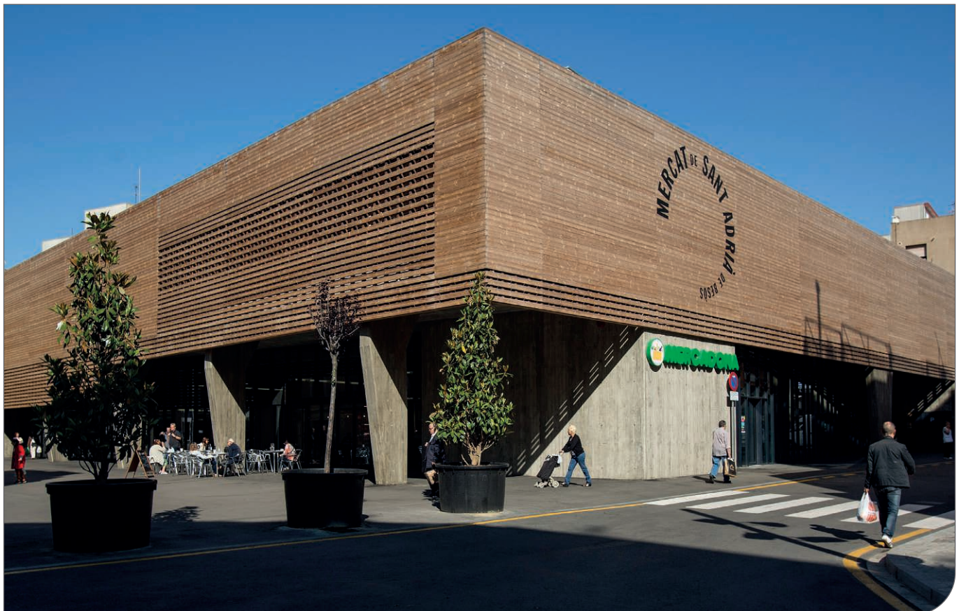
Figure 63. ThermoWood® exterior wall cladding on a Spanish shopping centre.
